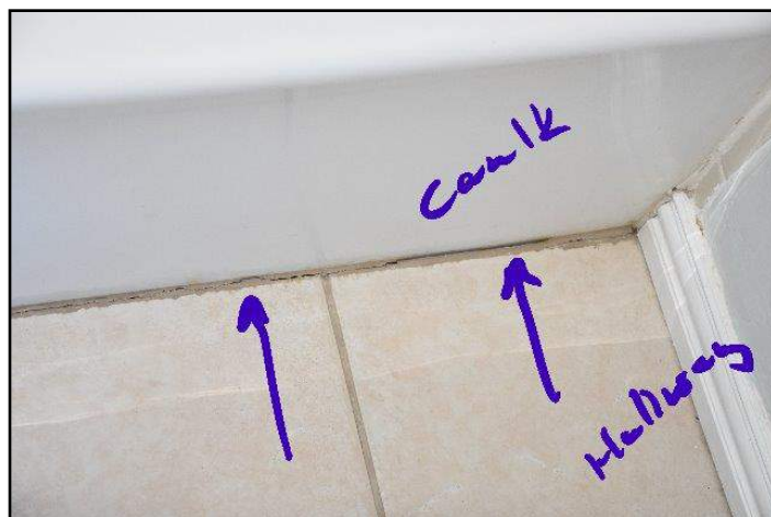
97. Caulk Tub and Tile interface water entry...
