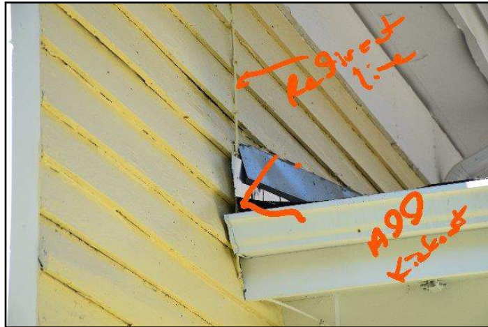
10. Kickout flashing - missing
