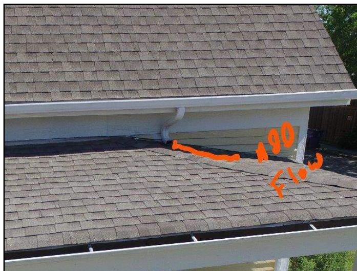
11. Discharge onto roofs
