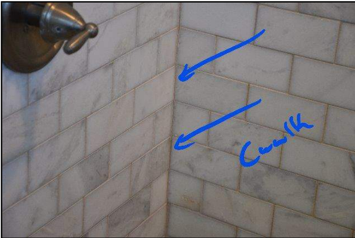
103. Caulking loose, missing or deteriorated
