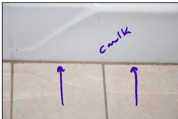
99. Caulk Tub and Tile interface water entry...
