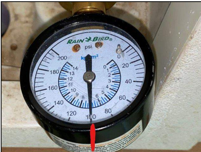
86. Recommended due to high supply water...
