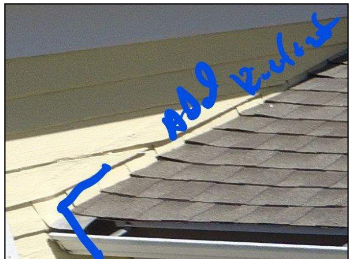
9. Kickout flashing - missing
