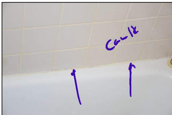
96. Caulk Tub and Tile interface water entry...
