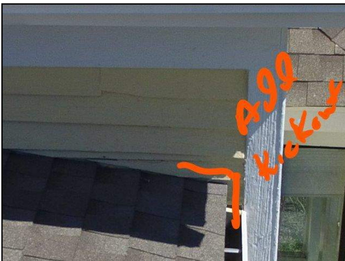
8. Kickout flashing - missing
