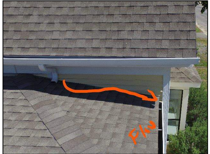
6. Roof Siding/Trim min 1" from Shingles. This...
