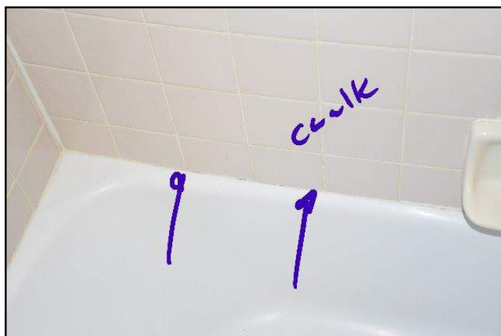
98. Caulk Tub and Tile interface water entry...
