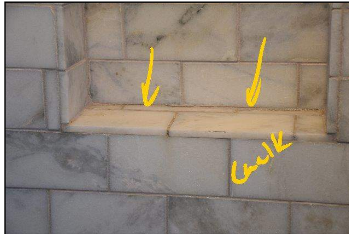
105. Caulking loose, missing or deteriorated
