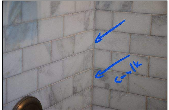
104. Caulking loose, missing or deteriorated
