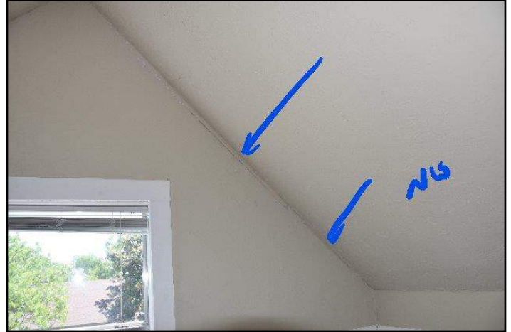
112. Minor Settlement Cracks
