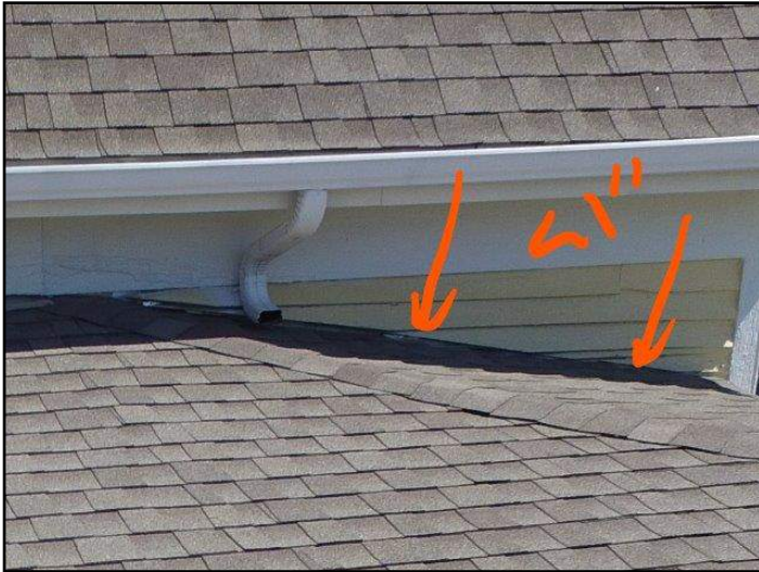
5. Roof Siding/Trim min 1" from Shingles. This...
