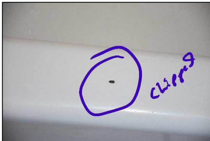
95. Cast Iron Tub Chipped
