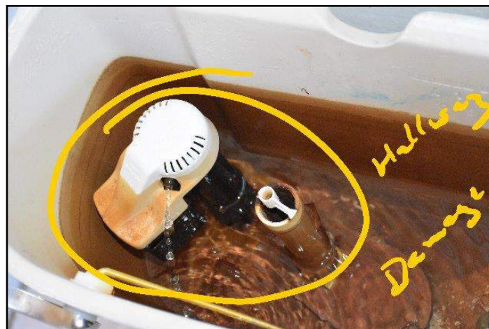
106. Flush mechanism inoperative
