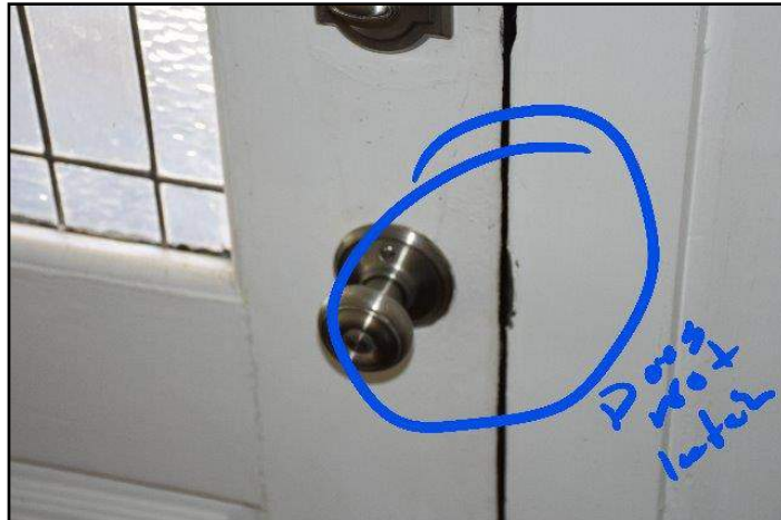
117. Latch not effective on exterior door
