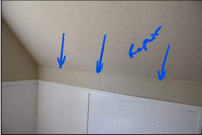
111. Minor Settlement Cracks
